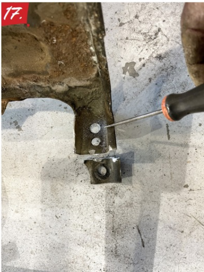
17. Harrison drills a second hole to achieve better stability once the battery tray is in place.
