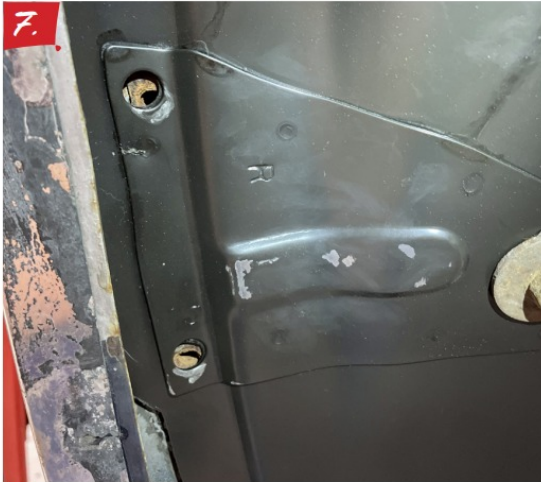
7. The reinforcement brace will need to be opened to line up the bolt holes. A stubby step bit works great for this. The holes aren't off very far.
